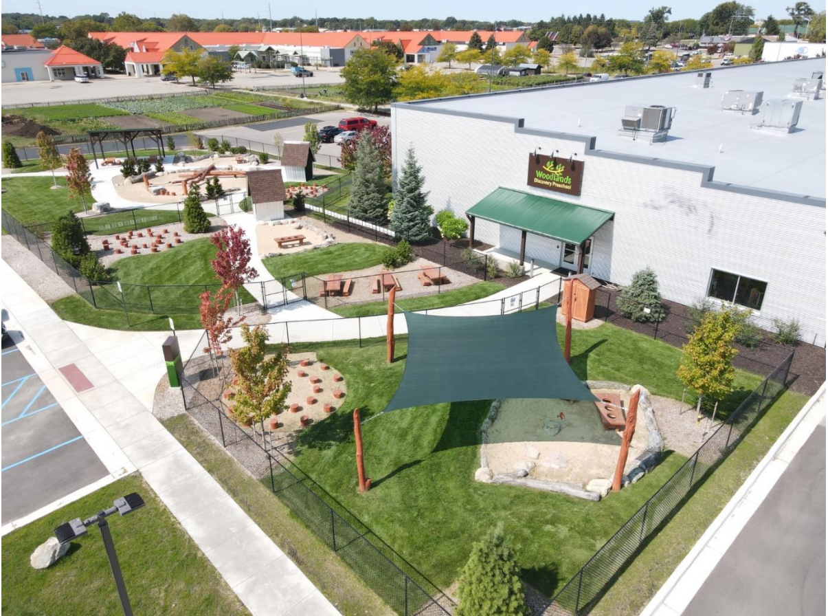
Strip mall redeveloped into nature-based child care center. Courtesy of Outdoor Discovery Center
