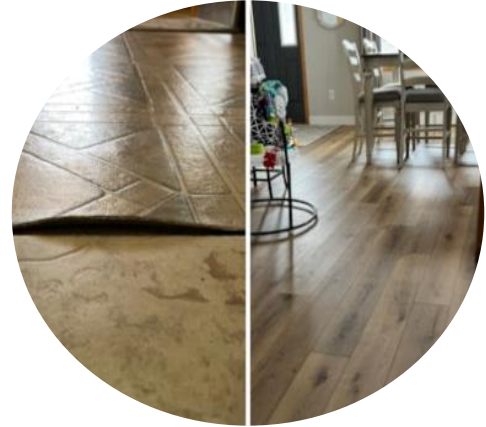
Damaged flooring replaced. Courtesy of FCF
