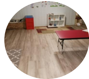
Replaced flooring. Courtesy of FCF
